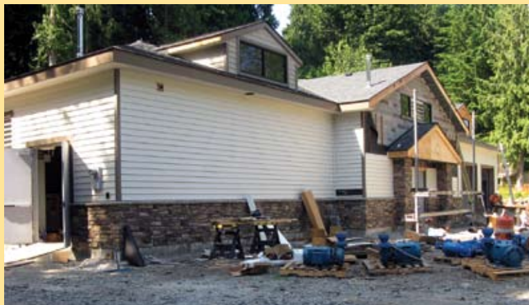
Construction at the new treatment facility is nearing completion.
