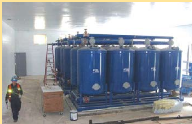
Twenty four filter tanks were installed inside the new treatment facility.
