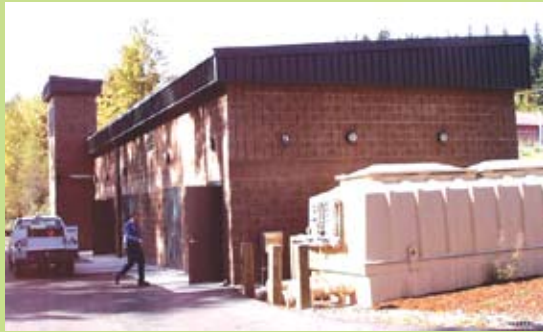
Inglewood Lift Station
